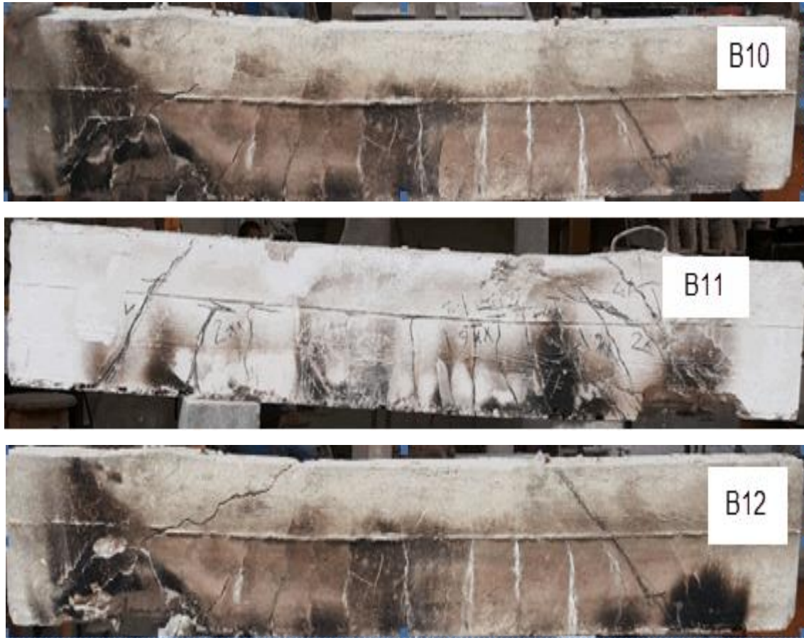
Fig (9): The Crack Patterns for Group 4
